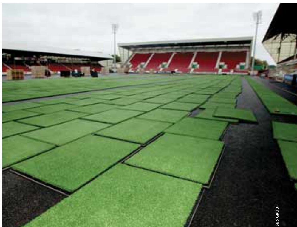
This jigsaw puzzle was assembled into the artificial pitch at East End Park, Dunfermline in 2003. The SPL had the artificial pitch replaced in 2005.
